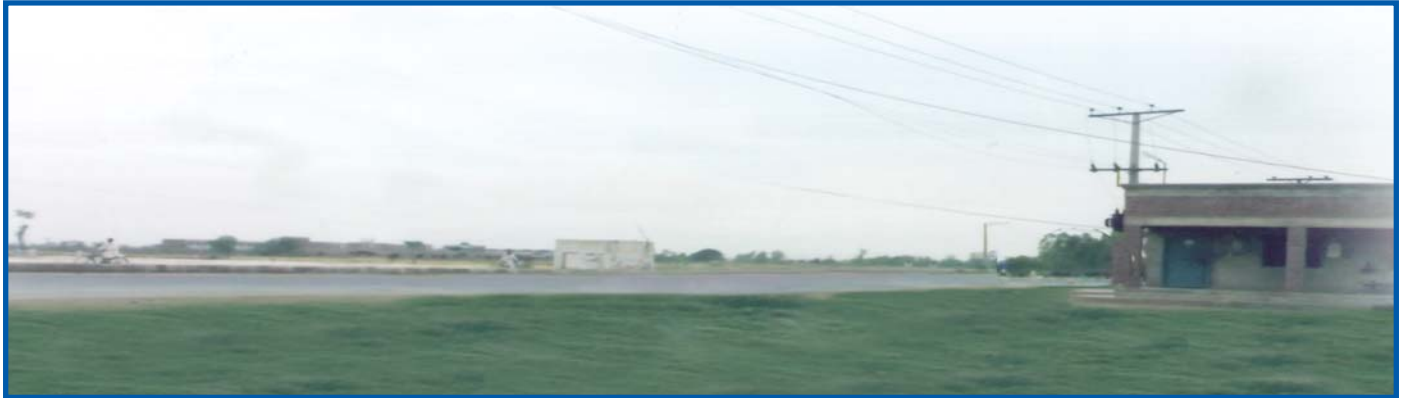
Proposed Site at Balochni, 40km from Faisalabad for establishment of Primary Health & MCH Center with Free Ultrasound
